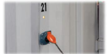
The display light of the identified socket starts blinking. The user can plug his battery to the socket.
