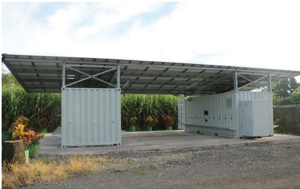
The framework of 100 m<sup>2</sup> of the unit is galvanized and demountable. It has been sized to withstand the strong winds of the cyclonic zones as well as the heavy rain, high temperature and a saline environment. The structure supports photovoltaic panels that allows to generate decarbonated and renewable electrical energy.
